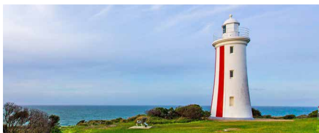
Mersey Bluff Lighthouse
